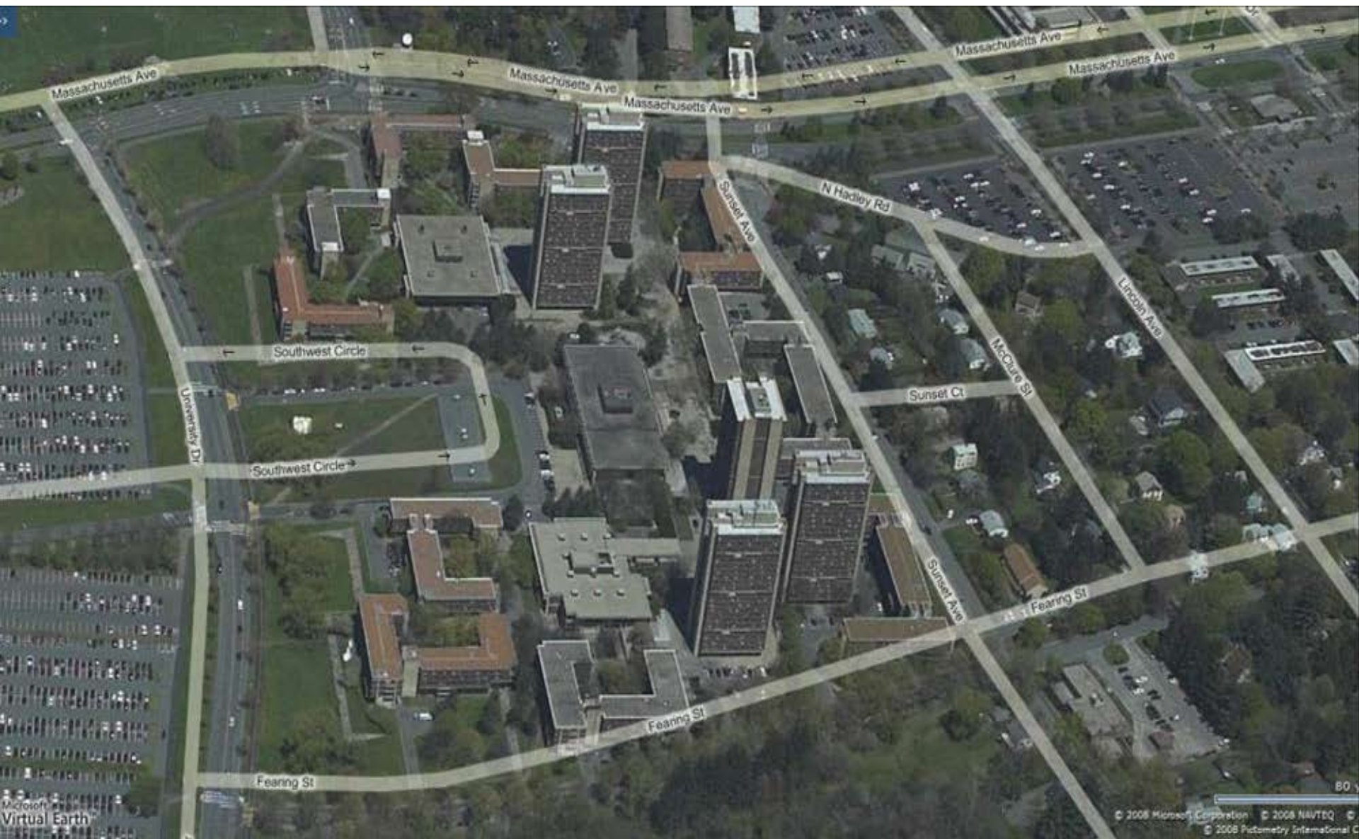
Aerial View Southwest Campus
